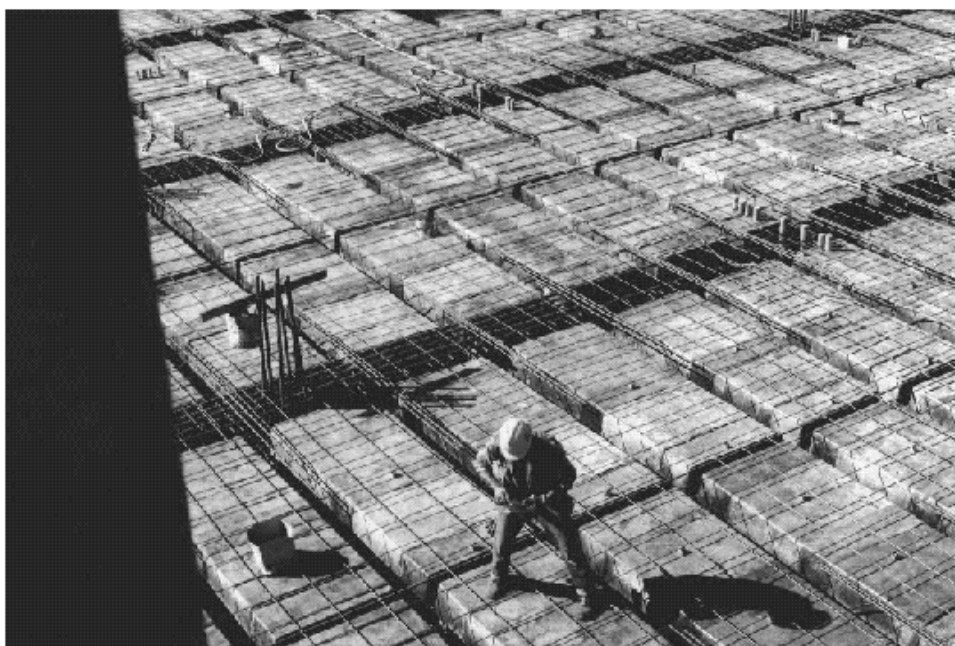
FIGURE 18.6 Steel forms for one-way joist floor.
