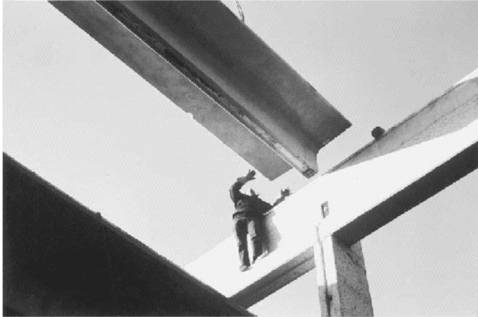
FIGURE 18.19 Long-span precast single T girder used with precast beams and columns.
