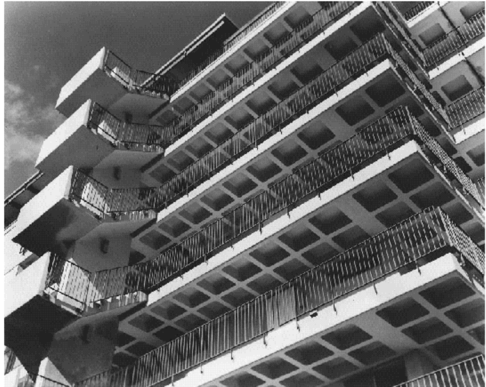
FIGURE 18.12 Regency House Apartments, San Antonio, with cantilevered two-way joist slab plus integral beams on column lines.
