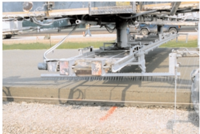
Fig. 11-20. Brooming provides a slip-resistant surface mainly used on exterior concrete. (69943)
