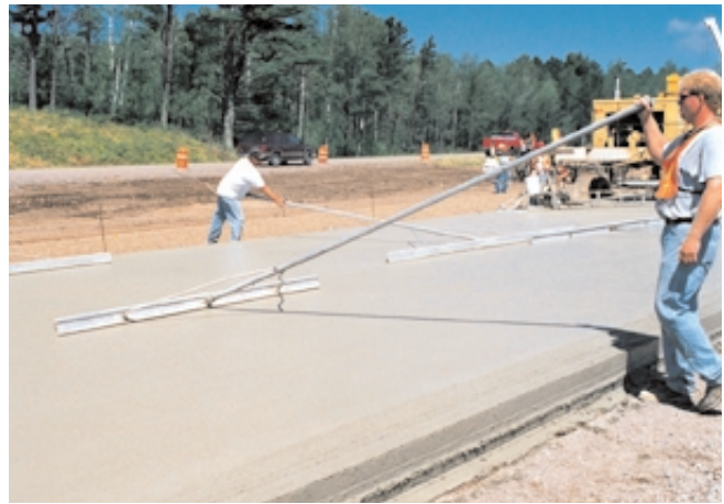
Fig. 11-17. Highway straightedges are used on highway pavement and floor construction where very flat surfaces are desired. (69941)
