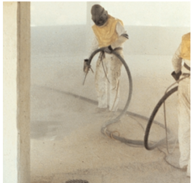
Fig. 11-23. Sandblasting can clean any size or shape surface – horizontal, vertical or overhead. Consult local environmental regulations regarding sandblasting. (55805)
