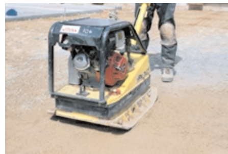
Fig. 11-3. (top) Adequate compaction of a base course foundation for concrete pavement can be achieved by using a vibratory roller. (bottom) Vibratory plate compactors are also used to prepare subgrades under slabs. (69934, 69930)
