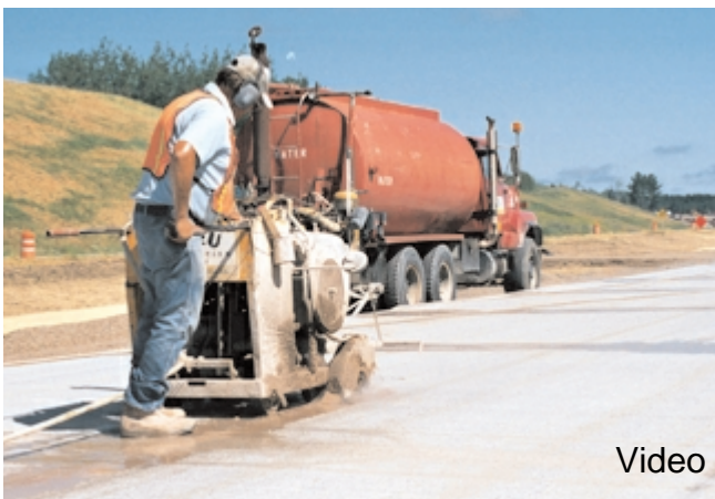
Fig. 11-28. Sawing a continuous cut in the top of a slab is one of the most economical methods for making a contraction joint. (69947)
