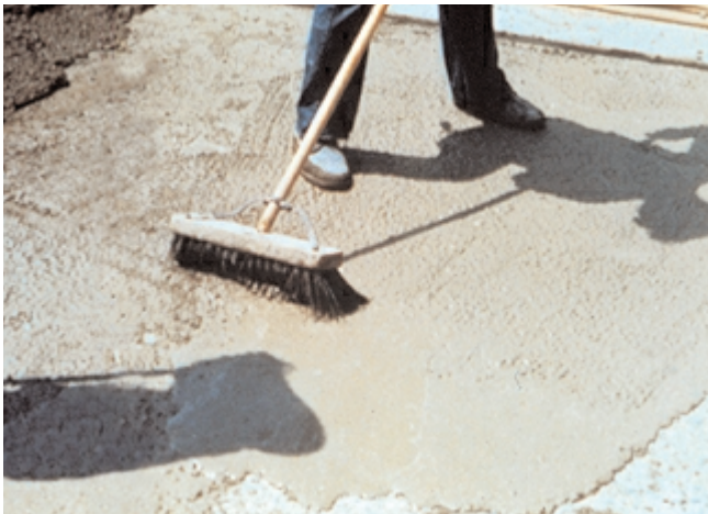
Fig. 11-25. Application of a bonding grout just ahead of the overlay concrete. The grout must not dry out before the concrete is placed. (51995)
