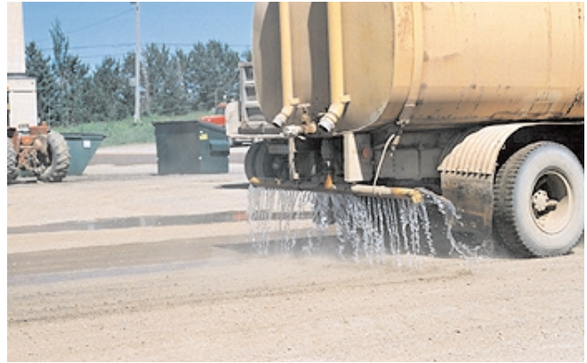
Fig. 11-2. Water trucks with spray-bars are used to moisten subgrades and base course layers to achieve adequate compaction and to reduce the amount of water drawn out of concrete as it's placed. (69931)
