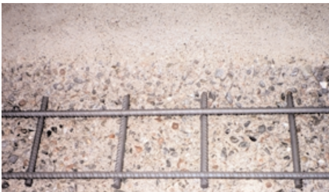
Fig. 11-32. Concrete prepared for patch installation. (69972)
