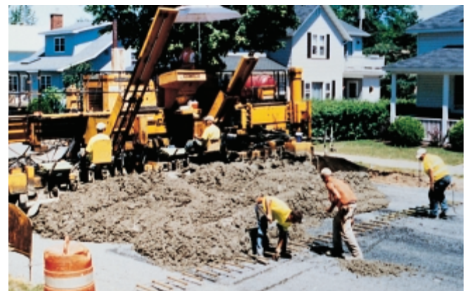
Fig. 11-6. Dump trucks deposit concrete ahead of a slip-form paver that places the entire width of a street in one pass. Epoxy coated dowels on metal chairs are positioned at a joint and spiked down to the base course just ahead of the paver. (69936)
