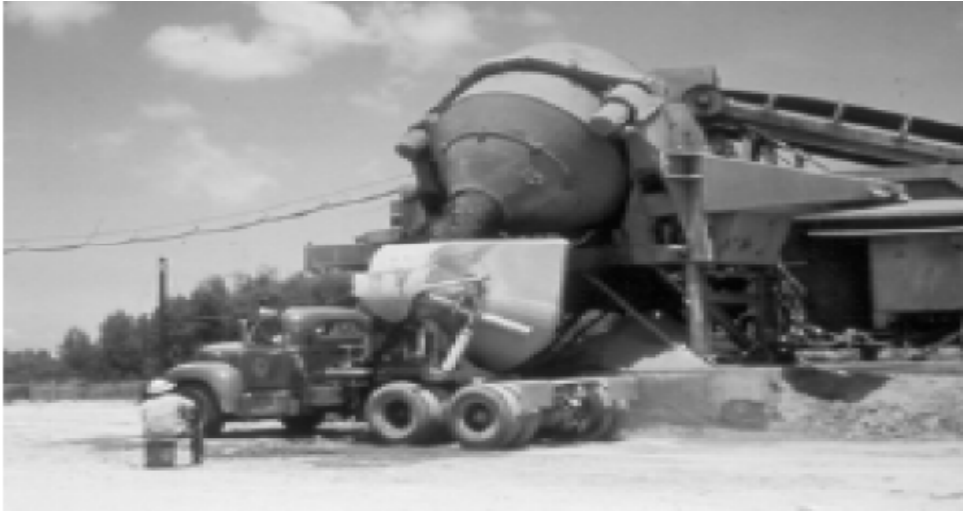
Concrete hopper truck at a concrete mixing plant
